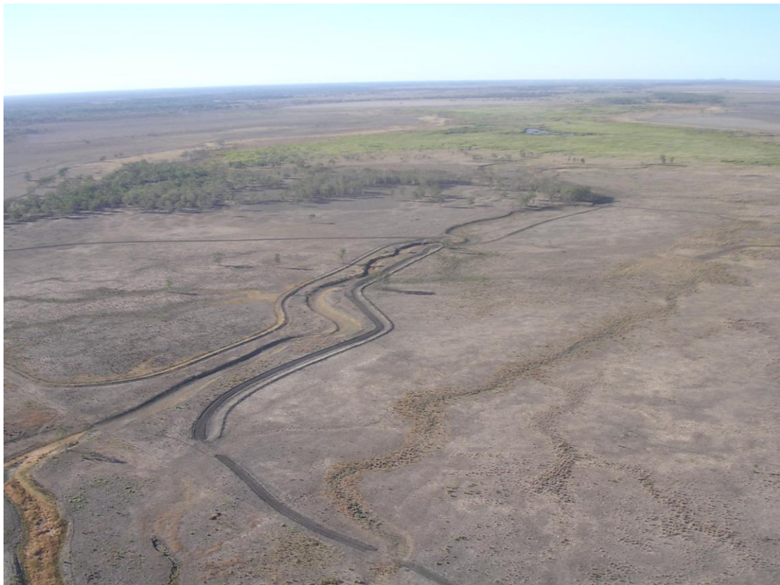
Photo showing banks being constructed upstream of the Northern Nature Reserve
